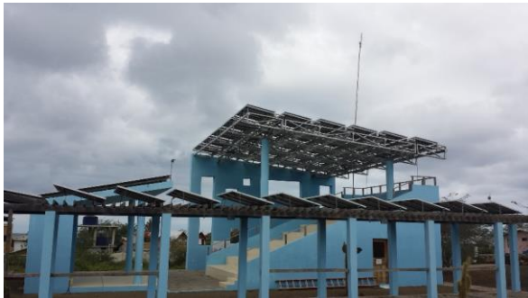
Fig. 16 Floreana solar PV power plant
