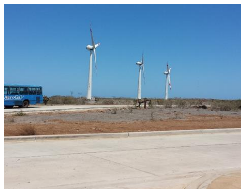
Fig. 12 Wind farm at Baltra
